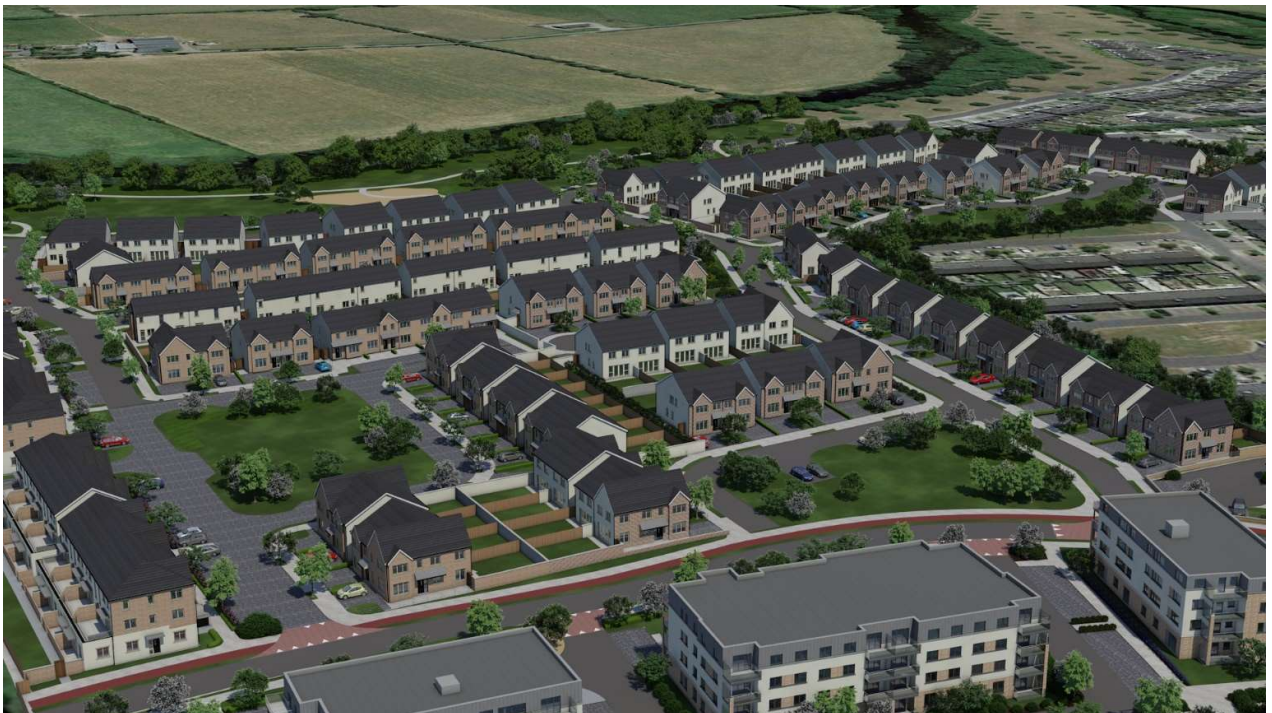
Fig 30: - Aerial View of the overall scheme from above the Brooklands Duplex blocks – Revised landscaping plan now incorporating the linear park along the river.
